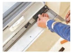
**Get the angle right.** Drywall returns rarely meet the window at 90°. Use a sliding T-bevel (also called a bevel gauge) to duplicate the actual angle.
