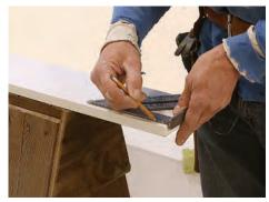
**Scribe the face cut.** Mark the depths taken from the window on the T-bevel lines, then use a square to mark where the horns will meet the wall.
