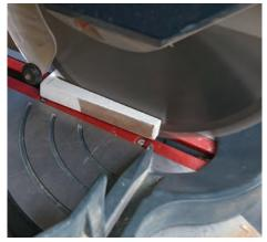
**Cut to the line.** Angle a miter saw to match the T-bevel line, then make a stopped cut up to the line where the horns will meet the face of the wall. Use a Japanese pull saw to finish the miter-saw cut and to make the rip cuts for the horns.
