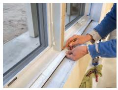
**Work from the center.** Use site-made pinch sticks to get an accurate measurement of the opening between the jambs, marking the window center on the strips.
