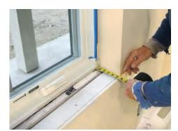
**Find the depth.** Measure from the window frame to the corner of the drywall. Check each side—the depths will sometimes differ.
