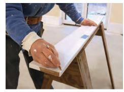
Mark the horns. Cut the stool 2 in. longer than the opening to allow for the stool extensions, or "horns". Align the aluminum strips' center with the center of the stock, and mark where the horns begin.
