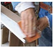
Sand for clearance. Properly cut, the stool will fit tightly. To avoid gouging the drywall, ease one bottom corner with sandpaper. Set the other end first, then drop the eased end into place.
