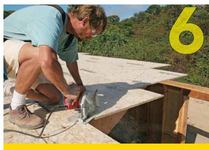
**ONLY MEASURE WHEN YOU NEED TO.** Tape measures are indispensable, but they can also introduce errors. Whenever possible, mark pieces in position rather than measuring them, and cut wall and roof sheathing in place during or after installation to improve accuracy.
