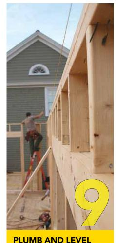
wall that is tipped into place should be rigged up with a string that runs from one end to the other so it can be pushed and/or pulled straight along its length. Although the method is different, joists, rafters, and beams must also be kept straight to ease the installation of the next pieces.
