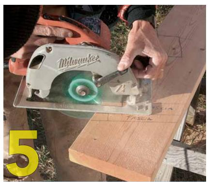
**AVOID GUESSWORK.** There's more to laying out framing than marking Xs for each stud position. Mark every wall component—kings, jacks, cripples, intersections, point-load posts, and blocking—to ensure you won't have to waste time later fixing inaccuracies. For complicated assemblies such as rafters or stringers, do a full-scale layout to avoid mistakes.
