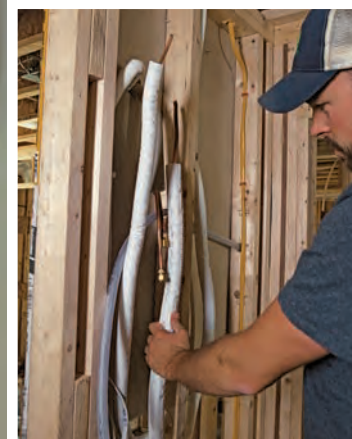
Minisplit heating and cooling. The line sets are run and the head units are installed before insulation takes place.
