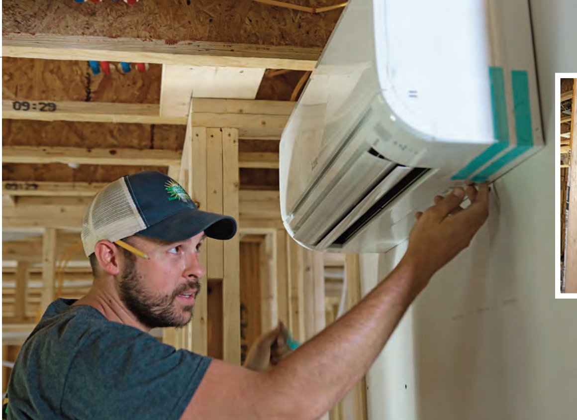
Minisplit heating and cooling. The line sets are run and the head units are installed before insulation takes place.
