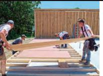
**Double-stud walls.** The exterior walls are framed on the ground and lifted into place. The inner walls are then framed in place.
