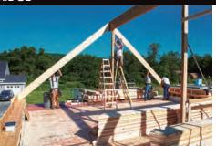
Structural ridge. Weyerhaeuser Eastern Parallam PSLs are used for the ridge beam and the posts carrying the roof load to the foundation.
