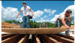
No-swell subflooring. AdvanTech subflooring stands up to the weather until the house is dried in. To eliminate squeaks, the subflooring is installed with AdvanTech subfloor adhesive on the top of the TJIs.
