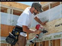
A hung floor. The floor joists are attached to a ledger on the inner wall. A strip of Intello Plus is installed behind the ledger to create a continuous air barrier.
