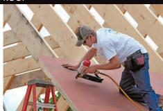
A quickly dried-in roof. Once the Zip System sheathing is nailed in place, the crew tapes the seams with Zip System tape and the roof is dried in.
