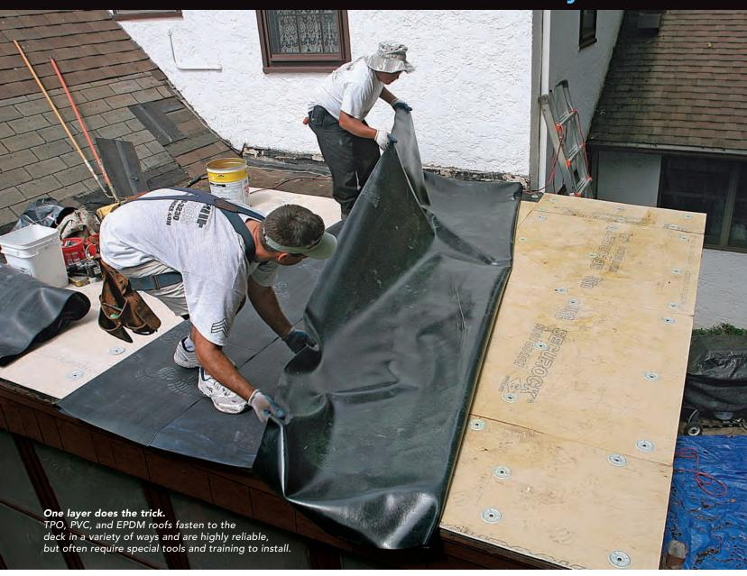
n cases where the roof is not subject to mechanical damage—say, by regular access required to maintain rooftop HVAC equipment—single-ply polymer-based membranes such as TPO, PVC, and EPDM are a terrific option. They are easy to clean, easy to inspect, and easy to repair in an emergency (although permanent repairs should be done by a professional certified in the manufacturer's
