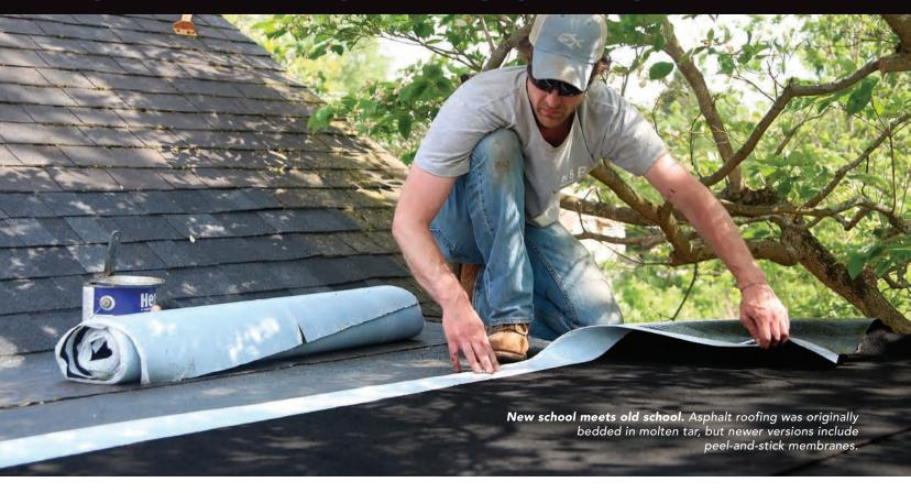
ost people are familiar with built-up asphalt roofing (BUR)—multiple plies of saturated felt or fabric applied shingle-style and layered with asphalt. The asphalt is melted in a big pot and pumped or bucketed to the roof and then mopped on. It is then covered with a cap sheet that has a mineral surface or a reflective coating (possibly acrylic, urethane, an asphalt-based emulsion—often with aluminum—or actual gravel carried up to the roof and spread by hand).
