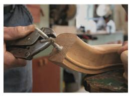
Insert the bolt. Eye the edge of a pair of locking pliers so they're even with the end of the rail. Align the bolt to leave room in the access hole to slip a wrench past, then clamp it tightly. Lube the treads with wax and turn the lag end into the volute. When the edge of the pliers hits the endgrain of the volute, the bolt will be at the right depth.
