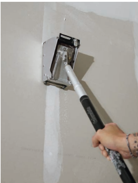
Spotters fill screws. Made in 2-in. and 3-in. widths, screw spotters are used to lay down a stripe of compound to cover drywall nails and screws.
