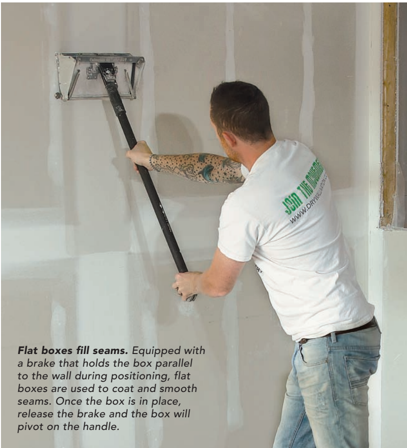
Adjust the flow. The eccentric cam adjusts the flow, so you can determine the amount of compound to dispense. The idea is to fully coat the seam without excess and leave a smooth finish free of voids as you go.
