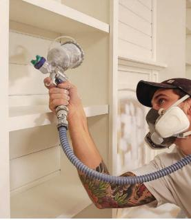
**Spot finish.** For blending and touch-up work, I set the air cap to the focused setting so I can limit my spray pattern to just the spot where I want it without creating a lot of overspray.
