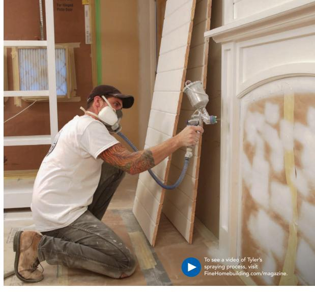
Finish flatwork in place. Relatively flat or open surfaces are less prone to blowback, so they can be leaned against a wall, set on a table, or installed and painted in place.
