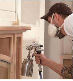
Seal with shellac. Waterborne primer will raise the grain on raw wood, so I start by applying two coats of thinned, dewaxed shellac to any stock that isn't factory primed, and to any spots where the factory primer was sanded through.
