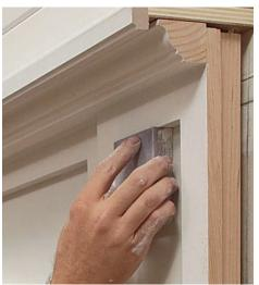
**Sponge sanding.** After priming, sand all surfaces to ensure a glass-smooth surface that's ready for top coats. I use a 150-grit sanding sponge, then I vacuum and use a tack cloth to pick up every bit of dust.
