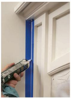
Caulk the transitions. Seams between components look best when sealed with caulk. After taping both sides of each joint, I apply Sherwin Williams SherMax and smooth it with a wet finger, then peel off the tape for a perfect bead.
