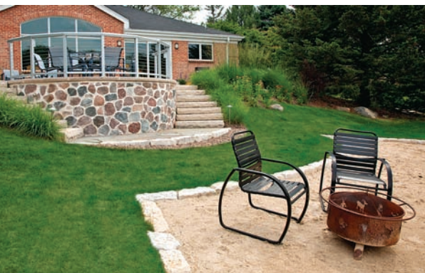
When to build a wall. A retaining wall creates a level area for the patio overlooking this steeply pitched lakeside landscape. Stairs wrap around the wall for access to the beach. Gardens surround the wall where the grade rolls away from the home.
