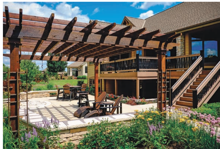
Style and shade. This cedar pergola defines a restful space within the patio. With an additional layer of purlins, this pergola blocks more sun than a common pergola. Trellises will direct vines to the top of the structure to eventually shade the patio even more.
