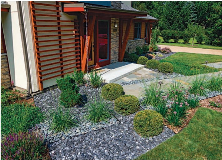
Rain, rain, go away. Rain gardens can be used to collect and direct water away from the house. Here, a rain chain acts as a gutter downspout and the pervious rock bed is pitched away from the home's foundation.
