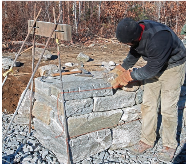
Build ends and corners like log cabins. Shaping is often needed to fit end stones. Alternate stones that span the wall width with long stones that tie back into each course.
