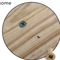
A small metal fixture breaks off the head of the screw, leaving only a tiny hole in the plank.
