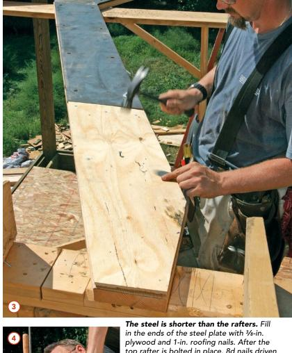
top rafter is bolted in place, 8d nails driven from each side will hold the tails together.
