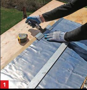
**Use hand-benders.** Mark the bend with a straightedge and a permanent marker, then turn up 1 in. of the first edge.
