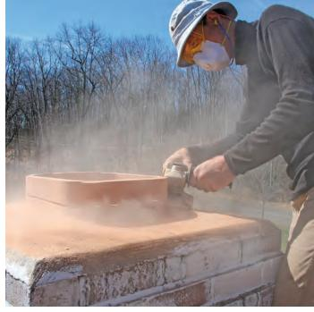
Parge the top. Mix successive batches of fastcuring mortar, and apply it in layers to fix damaged spots and create a smooth transition to the top of the flue.
