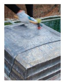
**Seat the lead.** Gently tap the lead sheet into the flue so that it laps down about ½ in.
