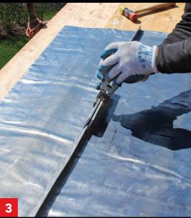
**Finish the seam.** Crimp the bends together, and fold them flat. Hammer them together with a series of light blows.
