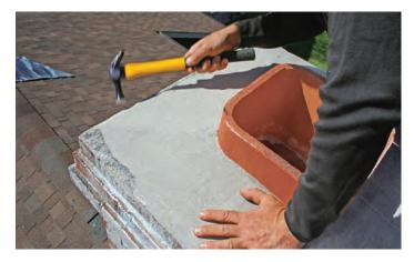
Cut the flue tile. Use an angle grinder with a diamond blade to cut back the existing flue, leaving it 1 in. higher than the surrounding concrete cap.
