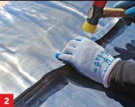
**Bend the second sheet.** Turn up 2 in. of the edge on the second sheet, and bend that over the first sheet's 1-in. up-turn.
