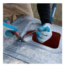
**Cut out the flue hole.** Use snips to make the cut, leaving about a ½ in. of lead inside the flue.
