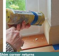
Shim corner returns square (photo left), and caulk the gap along the top (photo above).
