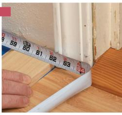
Eased edges of casing can be tough to measure to, so lay a block flat and measure to the edge.
