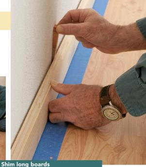
Longer boards spring into place for tight joints (photo left). Check them with a string, and shim them straight, if necessary (photo above).
