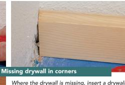
Where the drywall is missing, insert a drywall screw to keep the base plumb in the corner (photo left). Adjust the screw until it's even with the wall (photo above).
