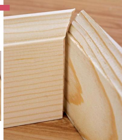
in the corner and the butt end of the coped piece slips into position.
