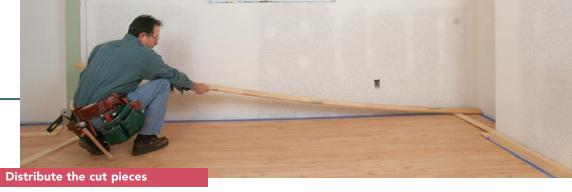
Place the lengths of baseboard around the room near where they are going to be installed.
