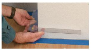
Outside corners aren't always 90°, so be sure to check the angle of the corner with a protractor.
