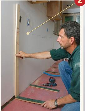
Due to the fluctuations in the subfloor, the plywood strips won't all be the same thickness. I rip 2-in.-wide strips of ¼-in., ½-in., and ¾-in. plywood and use a 34¼-in. gauge stick (the height of the cabinets less the countertop) to determine which size strip to use. I place strips at each end of a run of cabinets and anywhere cabinets are joined.
