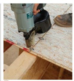
**5** Space the nails correctly. Drive the nails no farther apart than 6 in. on the short edges and 12 in. in the middle of the sheet, completely nailing each sheet before moving to the next one.
