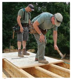
Tap gently. If the tongues and grooves in succeeding rows of sheathing don't engage easily, a few taps with a hammer against a 2x block should be enough to persuade them together.
