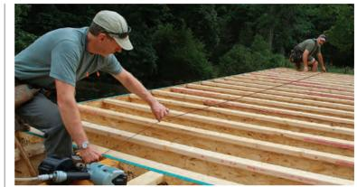
Start straight. Snap a chalkline across the joists 4 ft. from the outside of the rim joist.
