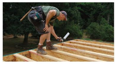
2 Start spreading the glue. Apply a bead of adhesive on each joist up to the chalkline.
