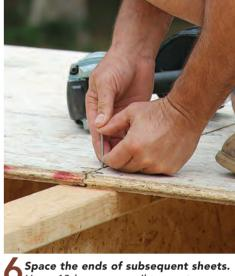
**Space the ends of subsequent sheets.**Use a 10d common nail to create an expansion space between sheets. After a few sheets, you may need to cut one shorter to keep the edges on the joists.
