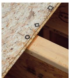
**3** Lay the first sheet. Align the edge with the chalkline. Choose either the tongue or the edge of the sheet; just be consistent.
