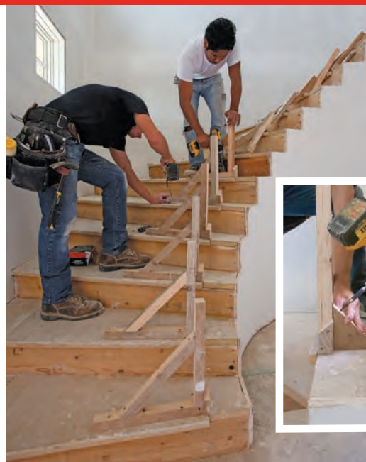
Bending brackets. Fastened 6 in. from the open end of each tread and parallel to the face of the risers, site-made brackets become the handrail bending form. The brackets at the upper and lower ends of the stairs are also braced laterally (inset) to resist the forces of the rail as it's pushed against the form.
