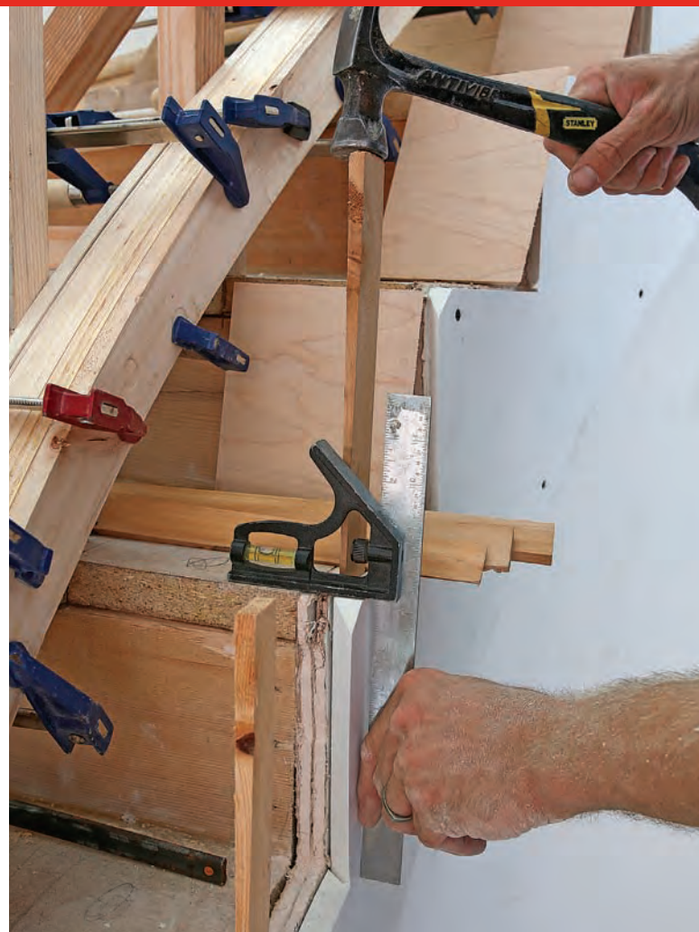
Shims for the win. To ensure a tight miter between the skirtboard and the riser stock, slide shims behind the skirt to square its face to the top of each rough tread.
