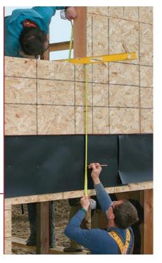
FIRST Adhesive-backed membrane applied to the wall sheathing protects the house by isolating the deck ledger. The membrane backing
