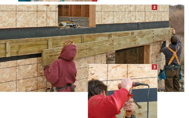
to the house with through-bolts and lag screws. The two-ledger system lets me attach the deck board nearest the house without perforating the flashing.
