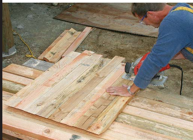
Third cut: Gang, mark, and cut to final length.
