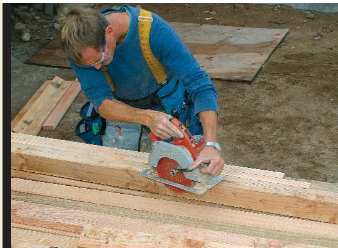
First cut: Make 70° tapered ends.
