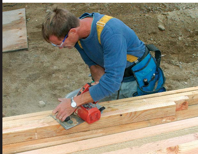
Second cut: Flip and cut through.
