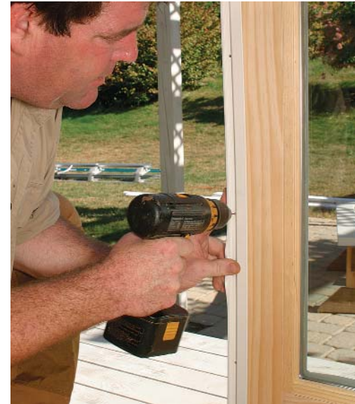
Weatherstripping goes where the two doors meet. Install the fixed-panel strip after this panel is in place. Make sure to orient the weatherstripping so that it will interlock correctly with its mate on the sliding panel.
