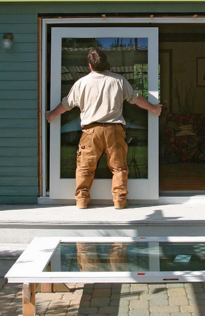
The fixed panel slips up, in, and down. After lifting it into place, push it firmly into final position against the side jamb.
