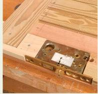
A lock mortise in layers. Simply making square cuts in the door's middle layer creates a mortise for the lockset. The hardware is located in the lower section of the door, where the paneling is installed.
