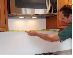
Test-fit the tiles on a flat surface. For the area above the stove, the author first measures the exact dimensions (top photo). Then he transfers them to a sheet of cardboard, where all the tile is dry-fit (bottom photo). Decorative elements such as the border and the square accent tiles are cut and fit at this time (photo left).
