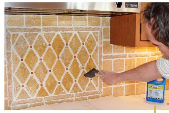
cleaning, I finish the job by applying sealer to the tile and grout. If the tile is stone (as in this case) and I sealed the tile before grouting, an additional coat of sealer also protects the grout. I apply the sealer with a disposable foam brush and give the backsplash behind the stove a couple of extra coats to protect the tile and grout from grease.  $\square$
