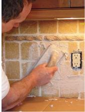
Seal. Grout. Seal again. Stone tile should be sealed before grouting to prevent the grout from sticking to it (photo left). After grout is applied and becomes firm, remove the excess with a sponge and dry cloth (photo right).
