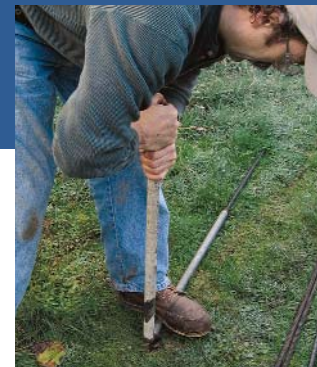
Bend to the desired angle.
