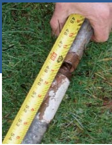
Put one pipe's opening at a corner.
