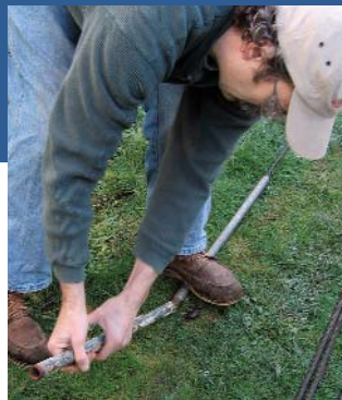
Slide the second pipe over.
