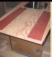
To support the weight of the island's cantilevered granite counter, carpenters routed broad cavities into the %-in.-thick plywood substrate, then screwed and glued two 1/4-in.-thick steel plates in place.
