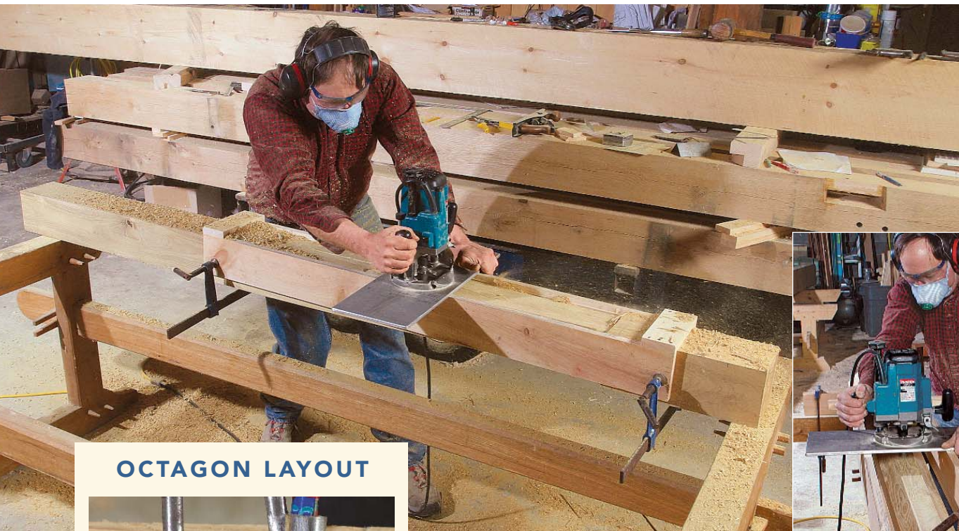
Flat sides are tapered first. A simple sled with the lower end elevated the depth of the taper guides a router equipped with a wide aluminum base for accuracy and stability.
