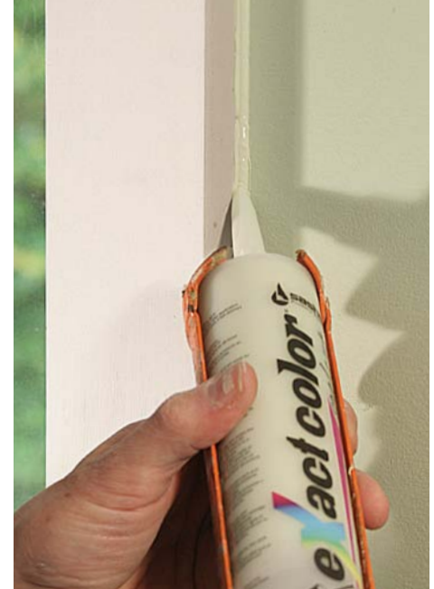
Caulk neatly. After allowing 30 minutes for the activator to thicken the caulk to a normal consistency, fill the joint.
