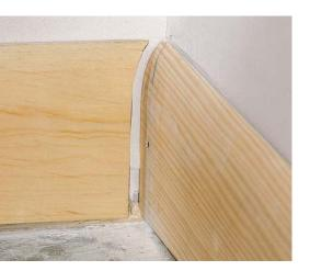
hen two pieces of trim meet at an inside corner, you could miter the joint, but most professional carpenters prefer to cope. An airtight coped joint is easier to produce: It doesn't require the perfectly square corner that a mitered joint needs. A coped joint is also less likely to open up after a few seasons of expansion and contraction.
