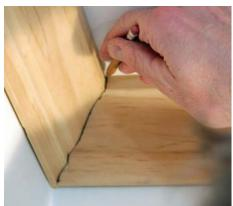
5 Close won't do. If the cope doesn't fit perfectly, a pencil serves to mark the high spots, which are removed easily with a rasp or some sandpaper.
