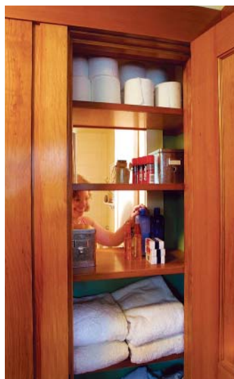
Smart and efficient storage. Open to both the bathroom interior and the hallway outside, a double-sided closet is used to store linens and supplies that might otherwise take up space in the small bathroom. Photo taken at G on floor plan.
