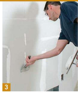
The butt seam is the most difficult seam to conceal. Taping leaves this seam slightly higher than the plane of the drywall. Spread compound in a 10-in.-wide band on each side of the seam, and blend the compound into the seam above 1. The trick is to fill in both sides without adding
