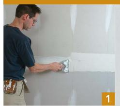
I usually don't sand between the first and second coats. But before applying the second coat of compound, I knock off any noticeable ridges or chunks of dried compound with the 6-in. taping knife.
