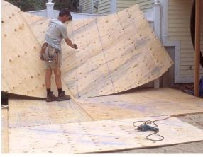
**Establish radius and treads.** Driven into the ground at a point in line with the upper landing, a stake becomes a pivot, anchoring the tape and chalkline used to draw the stair's shape and treads (photo above left).
