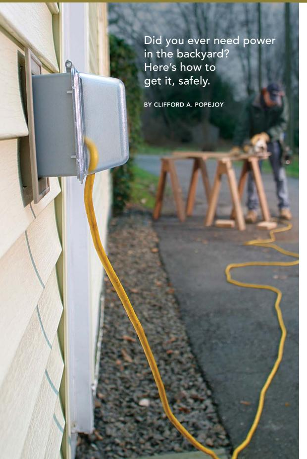
n most cases, adding a receptacle on the outside of a house is a straightforward bit of work. You locate the new exterior receptacle in the same stud bay as a general-use receptacle inside the house, cut an opening in the outside wall, fish cable from the existing electrical box to the new one, and make the connections.
