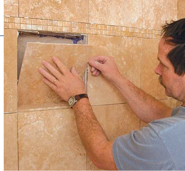
Starting with the bottom piece, line the recess with tile, followed in order by the back, top, and sides. All pieces should be back-coated with a layer of thinset.
