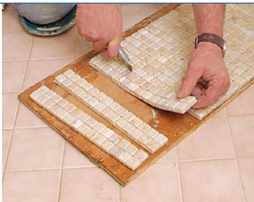
The next day, when the thinset has dried, the assembly is cut into uniform strips two tiles wide and to a length that matches the width of the large tiles.
