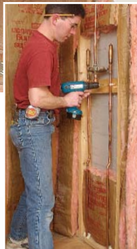
Time to call the plumber. The plumber levels the drain (photo above) so that it matches the shower-pan floor. He also replaces the mixing valve with a thermostatic pressure-balanced shower valve (photo right).
