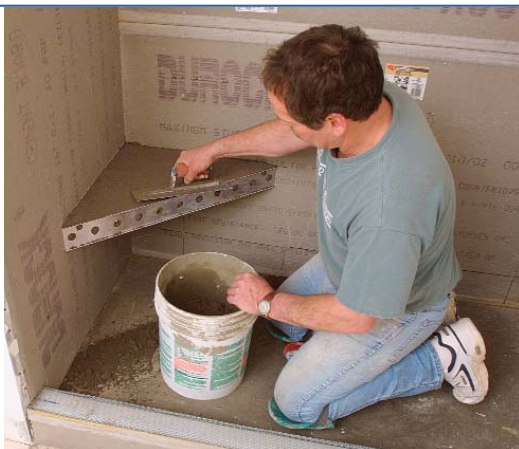
The form then is filled with mud that creates the substrate for the tile. After the top is leveled off, the mud is left to dry overnight.
