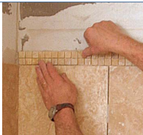
The strips now can be applied to the backerboard with a liberal coating of thinset.
