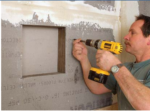
Remove the waste, then reinforce the opening with 2x scrap material secured to the backerboard with construction adhesive and galvanized screws.
