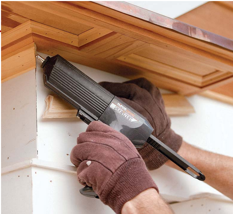
Permanent bond, almost instantly. A polyurethane hot-melt gun applies professional-strength glue that cures in as little as 30 seconds. A spring miter clamp ( www.right-tool.com ) draws the joint tight during the brief time it takes for the glue to cure.
