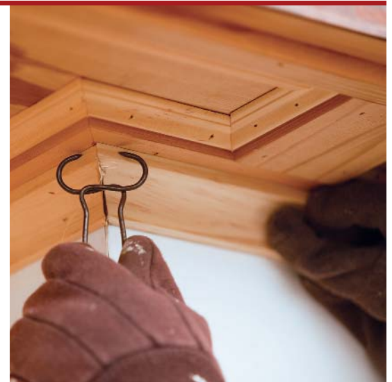
Permanent bond, almost instantly. A polyurethane hot-melt gun applies professional-strength glue that cures in as little as 30 seconds. A spring miter clamp ( www.right-tool.com ) draws the joint tight during the brief time it takes for the glue to cure.
