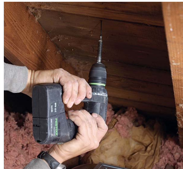
A screw marks the spot on the roof. A screw driven into the center of the traced circle and through the roof sheathing marks the center of the duct and transfers the vent location to the roof where the hole will be cut.
