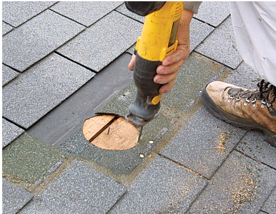
Cut a hole large enough for the vent. The hole for the vent should be slightly larger than the duct receptacle to allow the ductwork coming from the fan to slide into the sheathing and all the way onto the receptacle.
