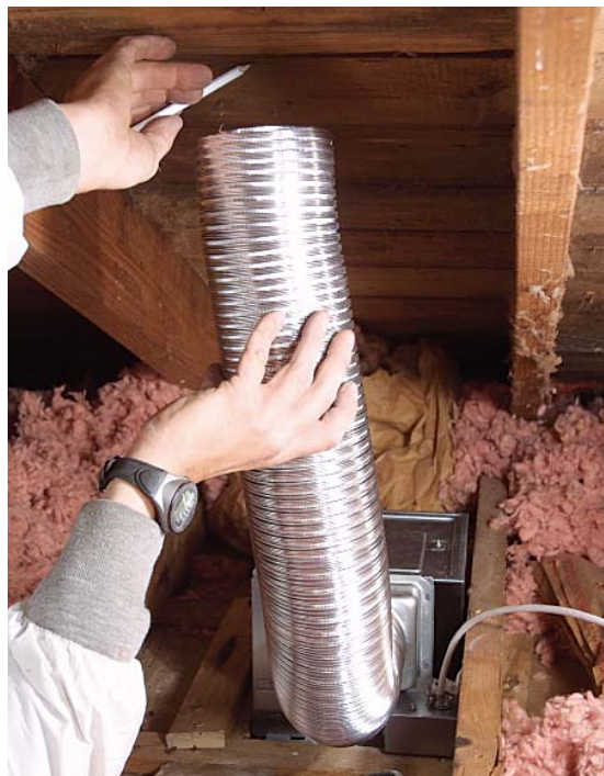
A screw marks the spot on the roof. A screw driven into the center of the traced circle and through the roof sheathing marks the center of the duct and transfers the vent location to the roof where the hole will be cut.
