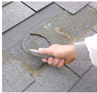
Cut a hole large enough for the vent. The hole for the vent should be slightly larger than the duct receptacle to allow the ductwork coming from the fan to slide into the sheathing and all the way onto the receptacle.
