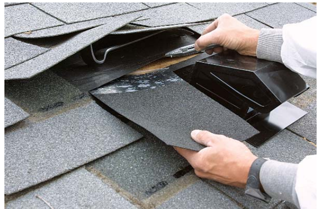
Overlap everything. A third piece of flashing, which also slips under the tar paper, overlaps the flange and the side flashing.
