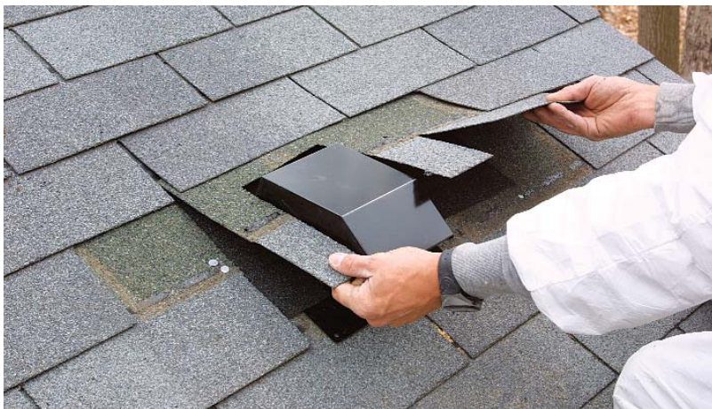
Cut around the vent and replace the shingles. Before the shingles are replaced, they are cut to fit closely around the vent, overlapping the flange on the top and both sides.
