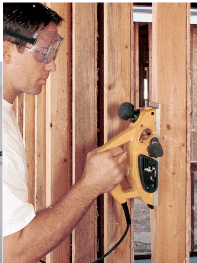
... straightening studs and other framing lumber
