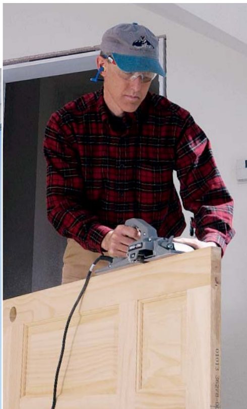
... fitting and beveling doors ...
