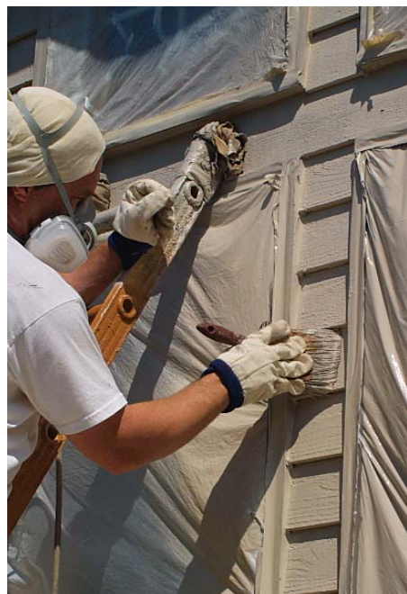
Siding is brushed after it's sprayed. With a spray gun in one hand and a paintbrush in the other, the author coats every surface that's comfortably within arm's length (photo left). Then he brushes to force the paint into all of the nooks and crannies (photo above).
