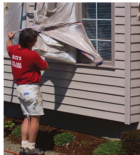
The moment of truth. As soon as the spray gun is unplugged, the masking is ready to come off. Pulling from the top down, the author gently removes tape and plastic to reveal smooth paint and crisp lines.
