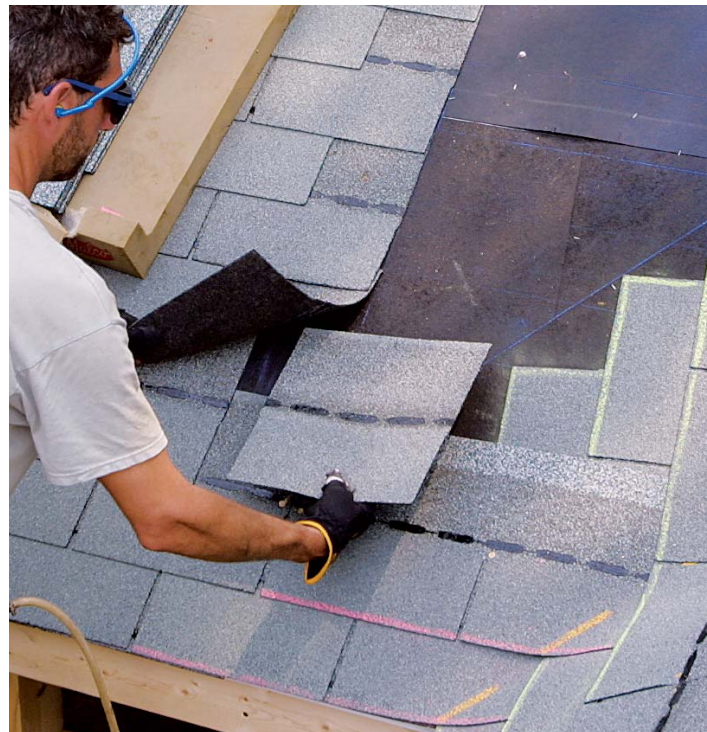
Insert a tab to stretch the course. Every course should wrap through the valley with a full shingle. A single- or a double-tab shingle may be installed to allow the shingle to extend through the valley (photo left) a minimum distance of 8 in., or the distance from thumb to middle finger (photo right).
