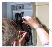
Mark the wires in place for accuracy. SER cable is heavy and stiff, so cutting the length and stripping the insulation accurately become critical.
