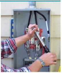
Loose connections can lead to fires. The right tools allow wire terminals to be tightened to the inch-pounds specified by the panel manufacturer.
