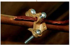
A bronze ground clamp bonds water pipes to the breaker-panel ground. Bonding draws current from accidentally electrified metal piping back to the panel, tripping the breaker.
