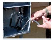
**Antioxidation paste** such as Noalox (www.idealindustries.com) keeps aluminum conductors from corroding.
