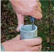
Reaming the cut end of metal conduit protects conductor insulation. Rigid-metal conduit for the service riser is cut to length with a metal-cutting reciprocating sawblade and then reamed to avoid damaging the conductor insulation.
