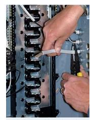
Label the cable. When the author rough-wires a house, he labels the outer jacket at the end of each cable with its circuit name. When tying into the panel, he strips the cable (leaving at least ¼ in. of jacket showing inside the panel) and places the labeled jacket over the hot wire to avoid later confusion.
