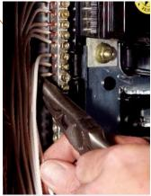
Tying in the neutrals. Needle-nose pliers help in tight spots. A torque screwdriver will tighten the terminal screws to specifications.
