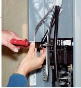
SER cable powers the breaker panel. The two hots and the white-striped neutral land on terminals just above the panel's main breaker. The bare ground locks in to the top of a ground bar. All are coated with antioxidant, just as at the meter base.
