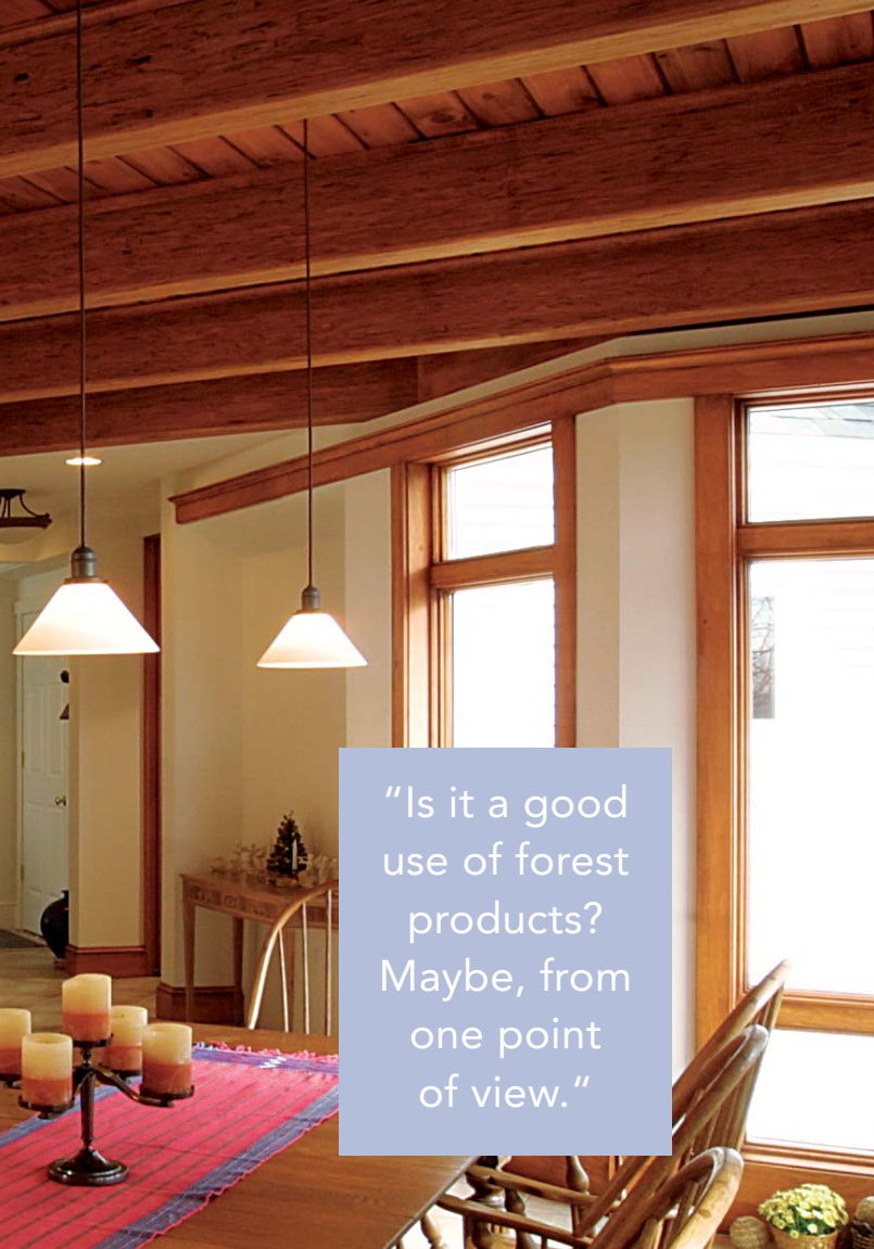
Exposed Parallam. A Connecticut builder liked the look of finished Parallam enough to leave the central girder and ceiling joists exposed in his dining room.
