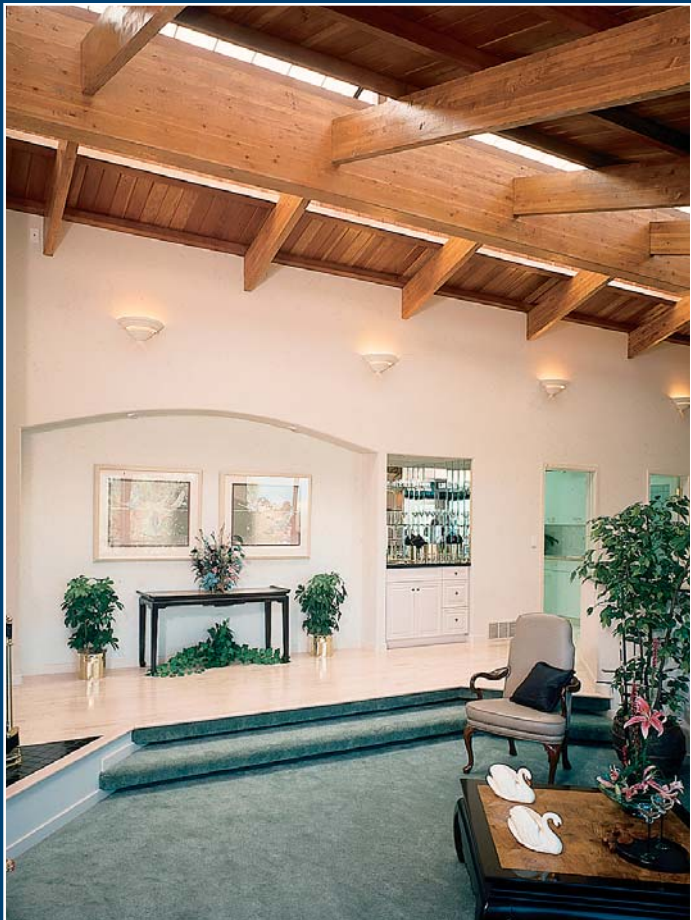
Glulam is a traditional choice for exposed framing. Rounded edges and a nice finish leave glulam looking good enough to use as an architectural feature.
