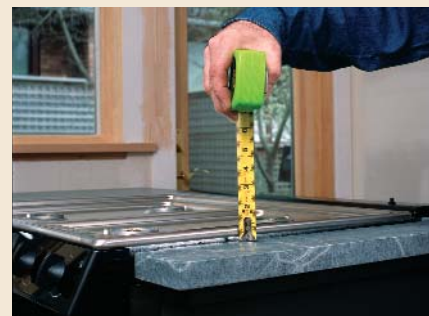
4. Don't scratch the countertop. Before positioning the range, extend leveling feet; lower them once the range is set.
