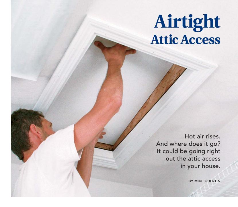
have been building airtight, energy-efficient homes for more than ten years. Before that, I built homes I thought were energy-efficient. Because I didn't make them airtight, though, I wasn't addressing half of the equation. Making a house airtight means closing the holes between conditioned spaces, such as the living room, and unconditioned spaces, such as the outdoors. I attack big holes first and work my way down until I reach the point of diminishing returns.
