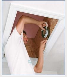
Inexpensive self-adhering foam weatherstripping works well and is readily available. However, it doesn't stick well to the edges of OSB or plywood. The author's solution is first to wrap the top edge of the shaft with aluminum duct tape and to apply the weatherstripping to that (drawing left). The weatherstripping sticks to the 1x2 cleats that support the lower hatch (photo above).
