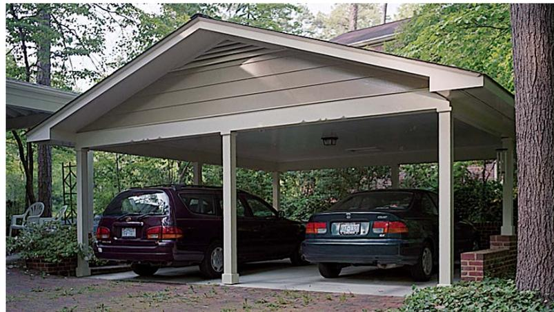
**Why doesn't it blow down?** It's easy to imagine a wind gust knocking over this structure that looks top heavy. Steel posts embedded in concrete and brick support the roof to stop that from happening.
