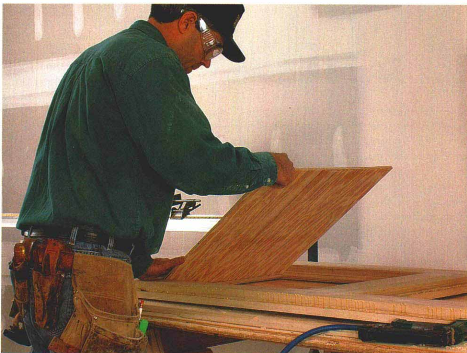
Beaded-plywood panel drops into place. Other panel styles—raised panels or tongue-and-groove boards, for example—easily can be substituted for plywood.
