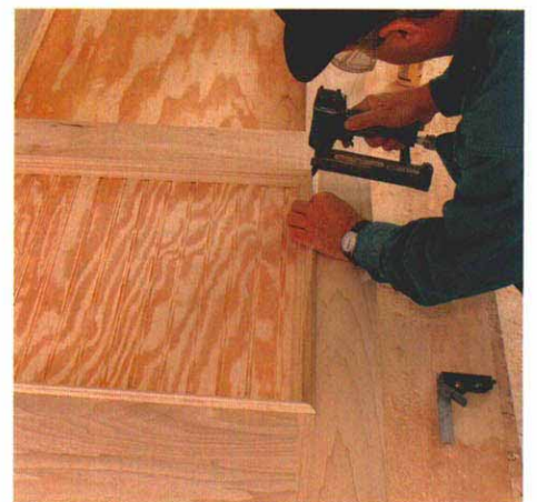
Additional face layer of molding is a Southern colonial touch. A flat panel and a simpler molding could give this door a Craftsman look. Whatever the molding, it holds in the upper glass panel as well.
