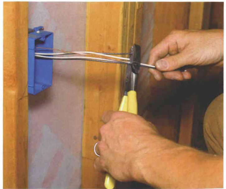
Side-cut pliers trim the conductors evenly.
