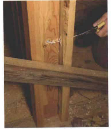
Going 'round the bend. After drilling intersecting holes, the author strips the cable to expose an easily maneuvered single wire. He works this wire around the turn and uses it to pull the cable.
