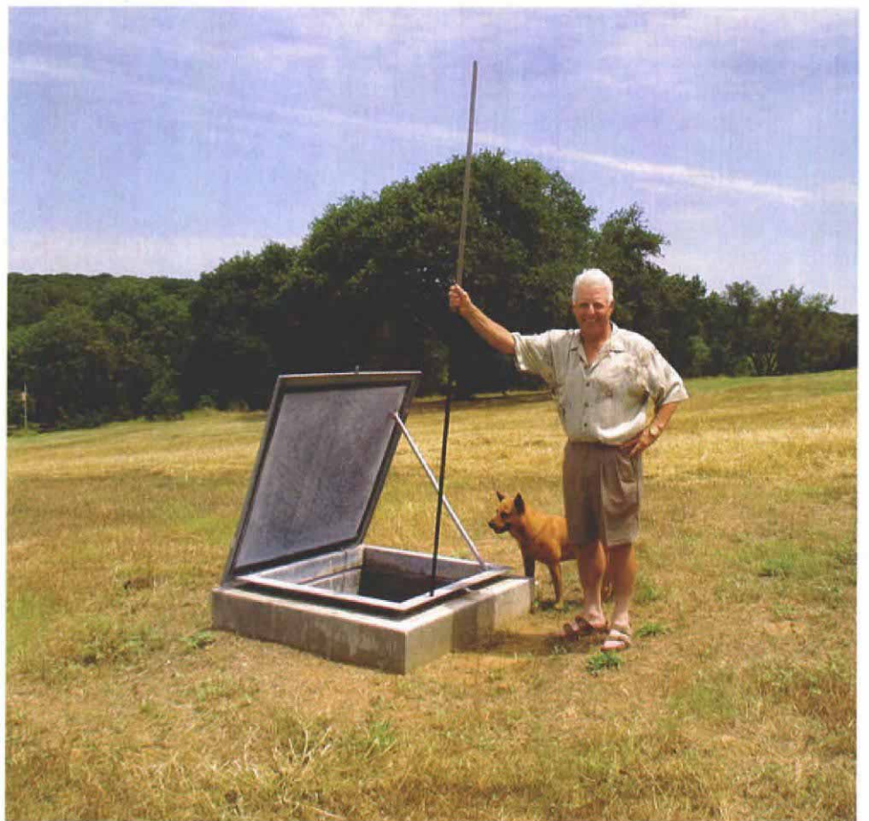
A big hole in one. The large flat cover of a cistern can be topped off with a patio or even a putting green (top photo). However, most cisterns are buried beneath the landscape with only the access hatch showing (bottom photo). Here, the owner and his dog use a long dipstick to check the water level in the 50,000-gal. cistern below the open hatch.
