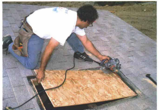
The sheathing is cut flush with the roof framing (photo above). Equal diagonals indicate a square curb (photo below).
