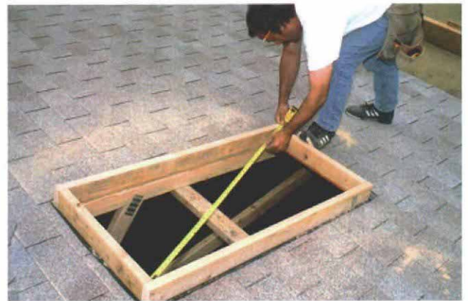
The sheathing is cut flush with the roof framing (photo above). Equal diagonals indicate a square curb (photo below).
