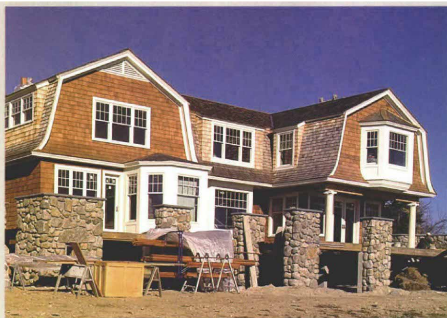
From agrarian to elegant. Gambrel roofs are used in barns to provide cheap space and to reduce rafter spans. In houses, gambrels add interest and allow a two-story home to have a relatively low roofline.
