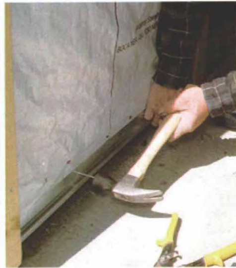
Bumping out the bottom. To get the siding started at the proper angle, a spacer should be installed behind the bottom edge of the bottom plank. A strip ripped from a plank (photo left) or galvanized Z-metal (photo center) can be used as a spacer.
