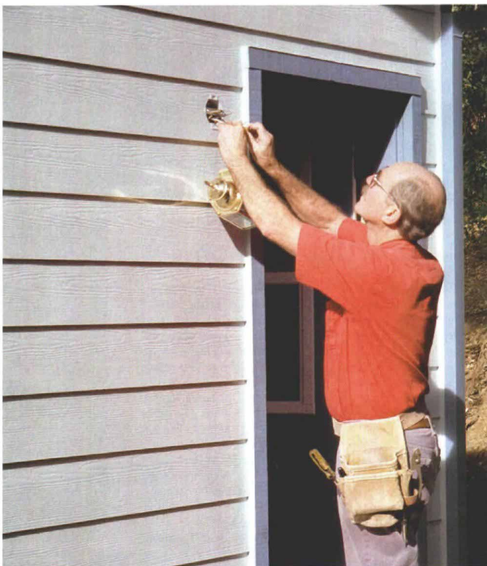
Primed and ready. Made of portland cement, sand and cellulose fiber, fiber-cement siding is resistant to all types of weather as well as insect damage, and it's fire-resistant to boot. The siding can be purchased primed, unprimed or with a finish coat of paint.
