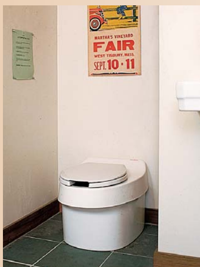
They don't look that different. To protect the aquifer on Martha's Vineyard, all the homes in the co-housing project have composting toilets.
