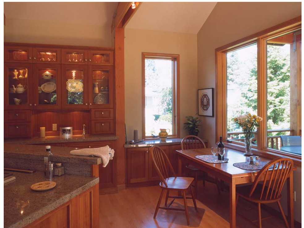
Built-in kitchen furniture. A beautiful cherry hutch is built between the posts of the central truss bay. Windows in the next bay light up the informal eating area. Photo taken at E on floor plan.
