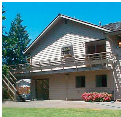
From flat to fancy. A covered porch on the kitchen addition (photo facing page) dresses up the original facade (photo above). Photos taken at A on floor plan.
